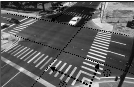
Two one-ways converge. Only one radii is correct (lower left). 1. Crosswalk is set back 25 feet due to wide radii. 2,3. Wide radii adds 2-3 seconds to crossing times (and adds to clearance interval and loss of cycle efficiency).
