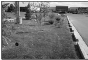
Parking lot sump
